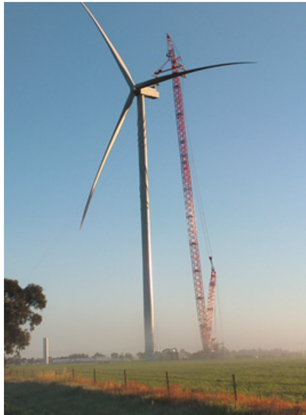
07 Installation of blade
