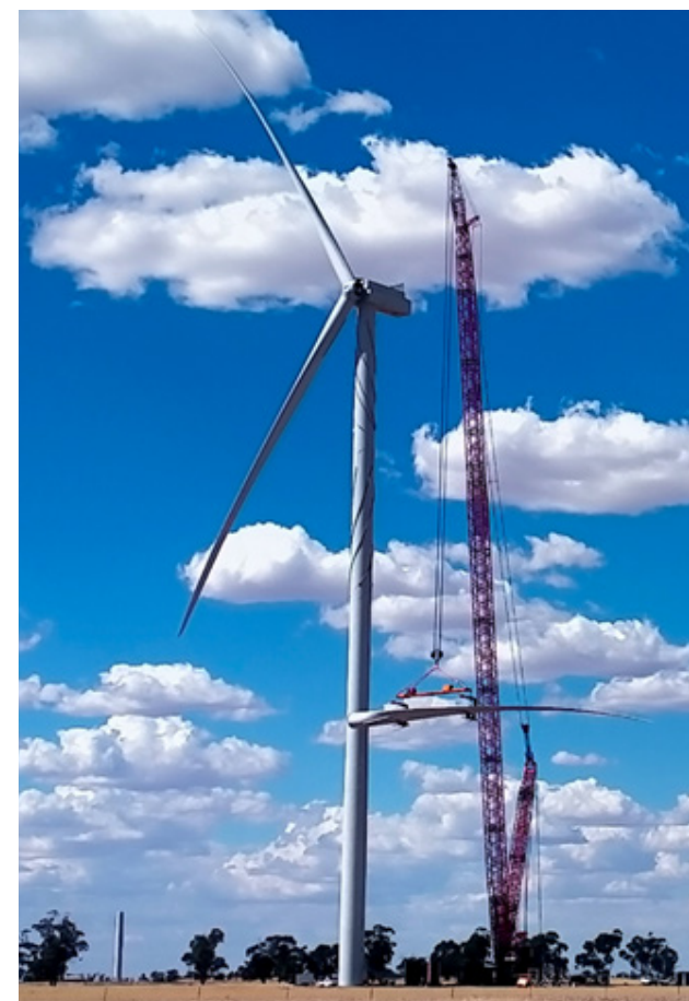
03 Installation of blade
